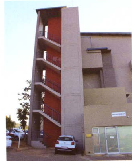
Included in the contract handled by J.C. van der Linde & Venter Projects was the installation of a new fire-escape.
