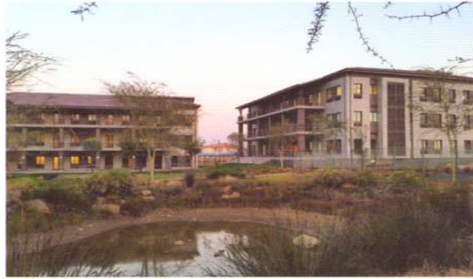
J.C. van der Linde & Venter Projects recently completed new additions to the Hazeldean Office Park development in Pretoria East.
